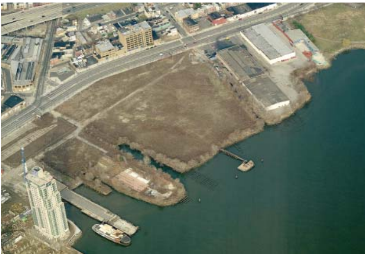
The proposed SugarHouse site, located in the northern portion of the project area
