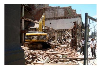
125. By late afternoon on the day before the collapse the front façade had been taken down, thus removing the only remaining lateral support for the wall.
