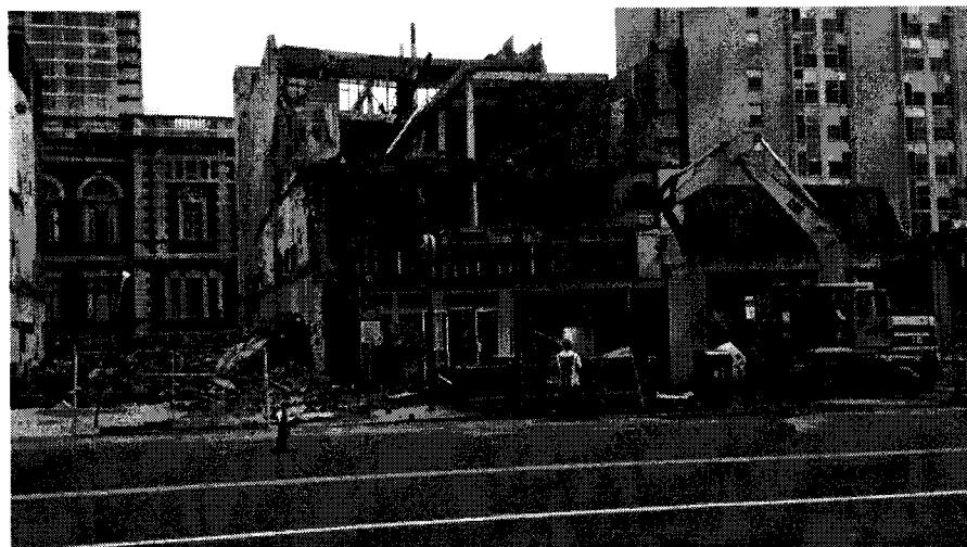
119. As these images show, Benschop used the excavator to demolish the front of the building by ripping out the floors, removing the lateral stability that the floors provided to the four story brick walls.
