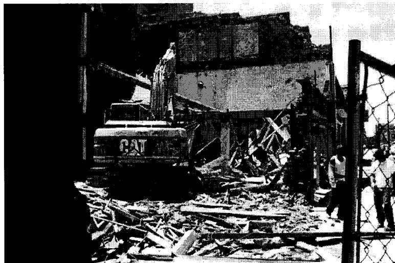
126. By late afternoon on the day before the collapse the front façade had been taken down, thus removing the only remaining lateral support for the wall.
